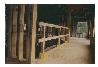
This Safety Boot Guardrail System (which includes toeboard slots), its construction and installation, meets OSHA regulations.
